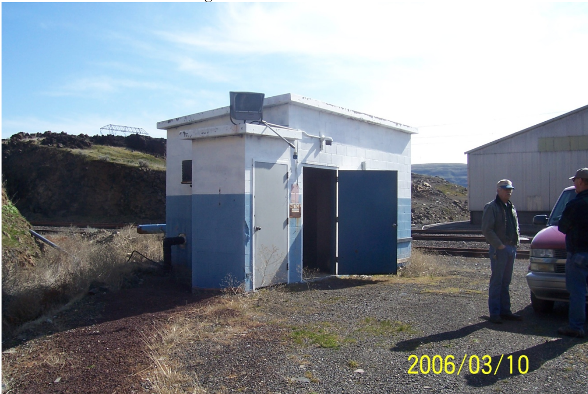
Picture 5-3 – Well No. 2 Building
