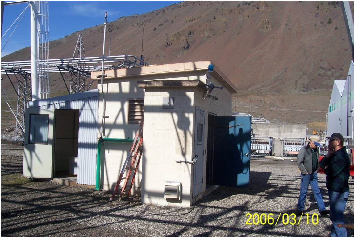
Picture 5-2 – Well No. 1 Building
