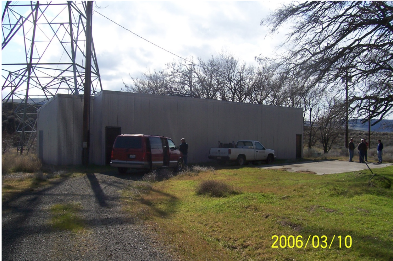
Picture 5-4 – Well No. 3 Building
