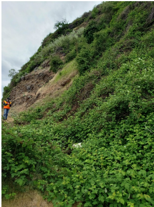
Photo 10: S24, Looking Southwest
