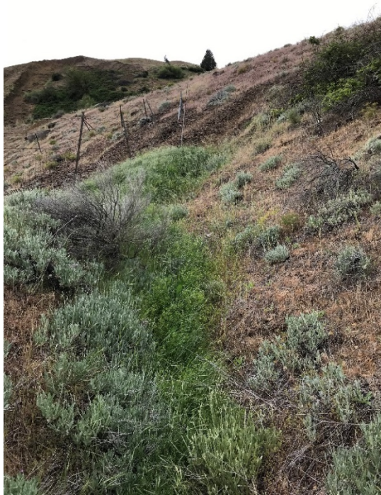
Photo 9: S17 at Culvert Outlet Located below Highway 14, Looking West
